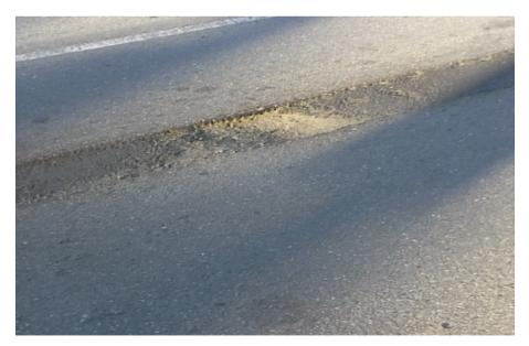
Utility companies that dig up streets have very little responsibility for the road after the trench has been patched up. It does not take very long for the asphalt to subside, leaving dangerous lips and potholes. And even when the patch does remain intact, the road surface often develops annoying undulations and bumps. In some cases, a considerable amount of money spent to stripe bikes lanes has gone to waste due to utility construction.
