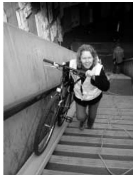
Laura Timothy, of BART's Customer Access Department, testing the prototype stair-channel
