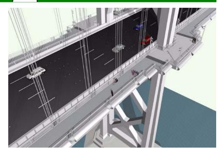
West Span Bicycle-Pedestrian-Maintenance Path would be cantilevered off both sides of the upper deck to complete the world-class bikeway all the way across the bay on the San Francisco side. Features of the path include benefits to motorists such as emergency vehicle access, refuge for stalled motorists, and reduced lane closures for bridge maintenance.
