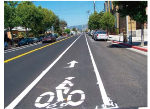
Emeryville's new Adeline Street bike lanes are a great example for traffic engineers everywhere to follow. Note that the curb-side (right) stripe of the wider bike lane is moved out and to the left, away from the "door zone" of parked cars. EBBC will work with Oakland and Berkeley to extend this "best" bikeway design to all five miles of Adeline Street, a major bike route.
