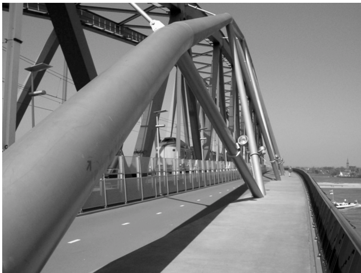
The Nijmegen railway bridge crosses the river Waal, in Holland. On the left, a passenger train can be seen crossing the bridge. On the right is a 770 foot long bike-ped bridge attached to the existing railway bridge in 2004.
