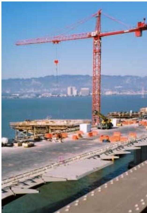
*View of new East Span under construction. The first decks of the Alex Zuckerman East Span Bikepath are attached to the support beams.*
