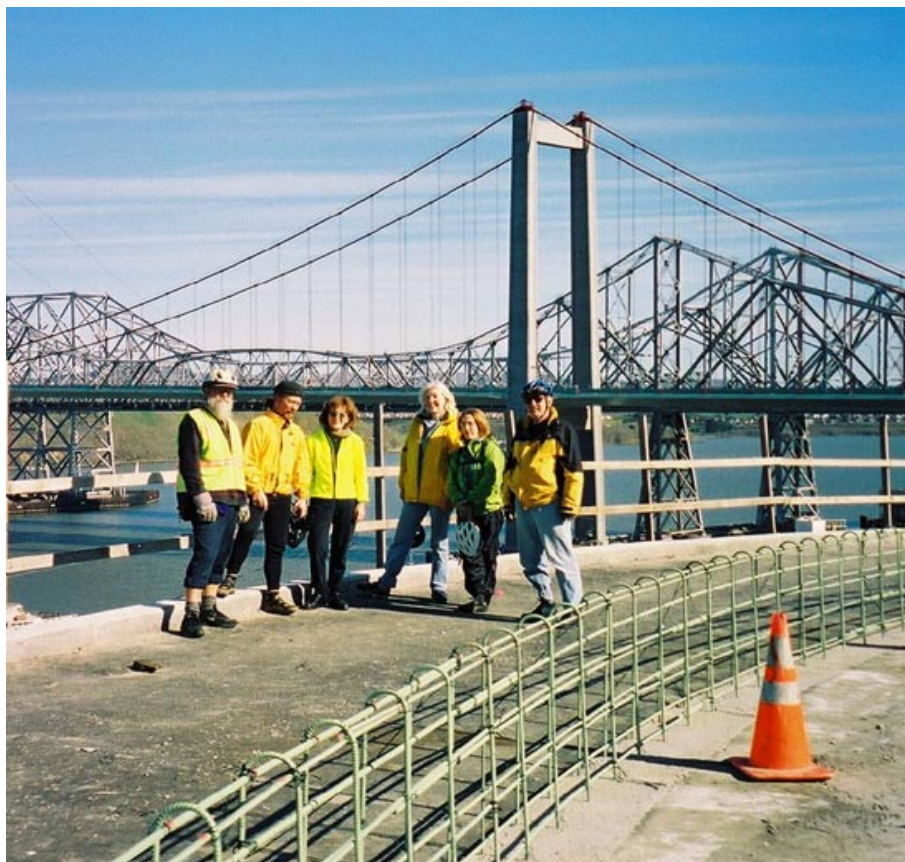
Following the annual retreat, a group of EBBC members inspect the approach to the Al Zampa Bridge Path from San Pablo Ave.. The structure is taking shape, but lacks guard rails and a barrier. The dedication of the facility will take place during Bike - to-Work week on Saturday, May 22 with Congressman George Miller. Mark your calendars!
